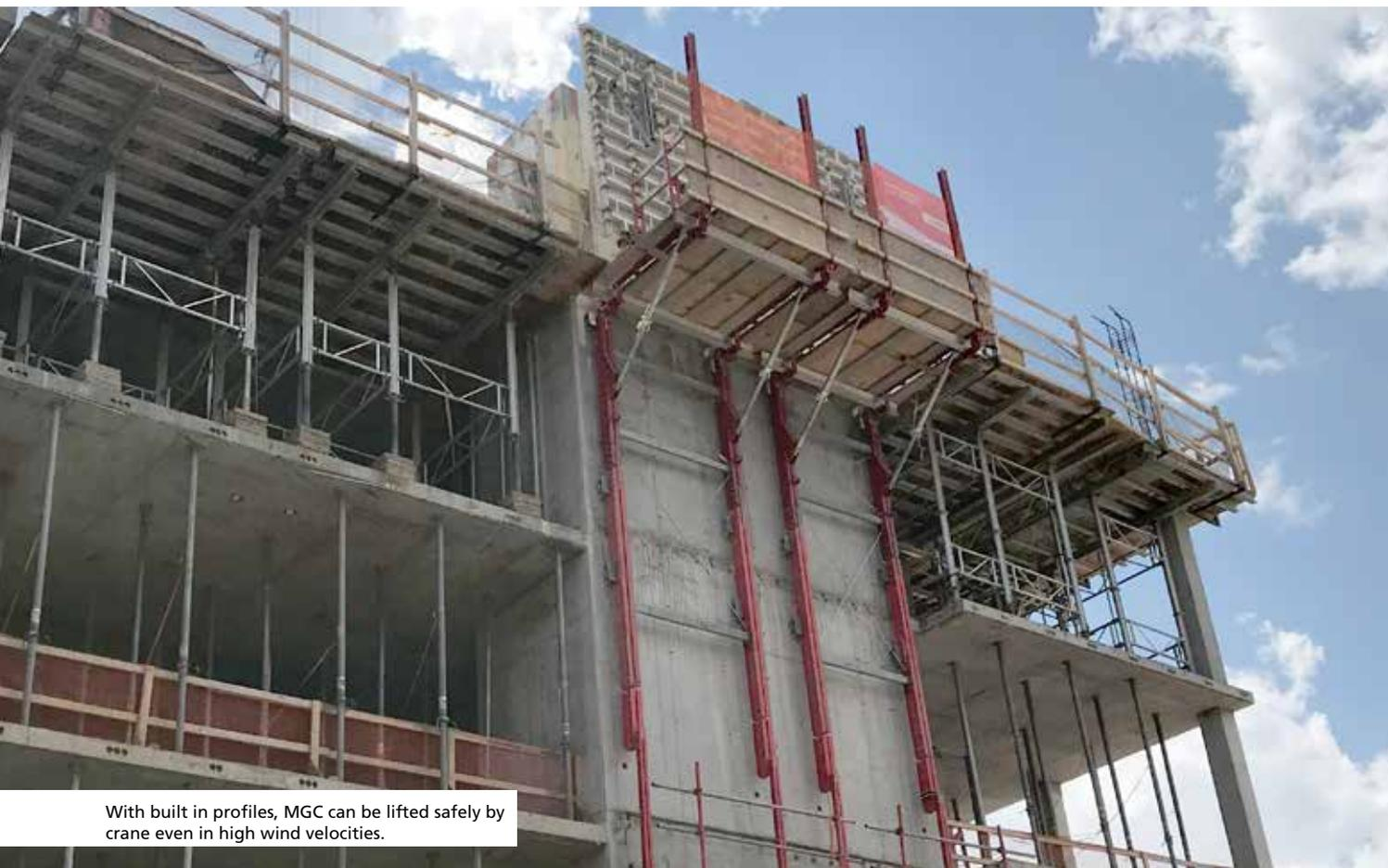
With built in profiles, MGC can be lifted safely by crane even in high wind velocities.
